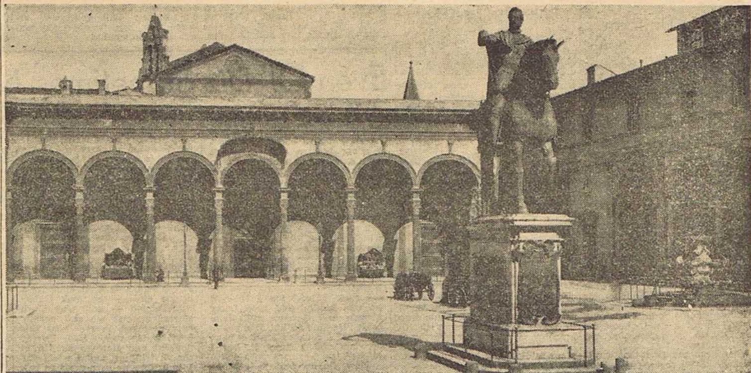
The Piazza Annunziata. In the background is the Church of the Annunziata with its portico done by A. Sangallo (1599-1600). To the right is the famous orphan asylum of Florence—first in Europe—limited to the legitimate offspring of the poor. The building is known for its terracotta lunettes of babies (between columns) by Andreas Della Robbia.
